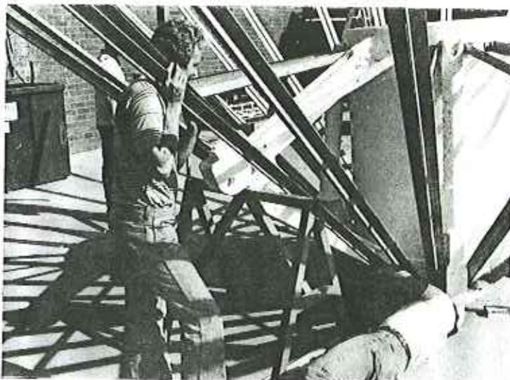
Install Radial Braces to Hub
