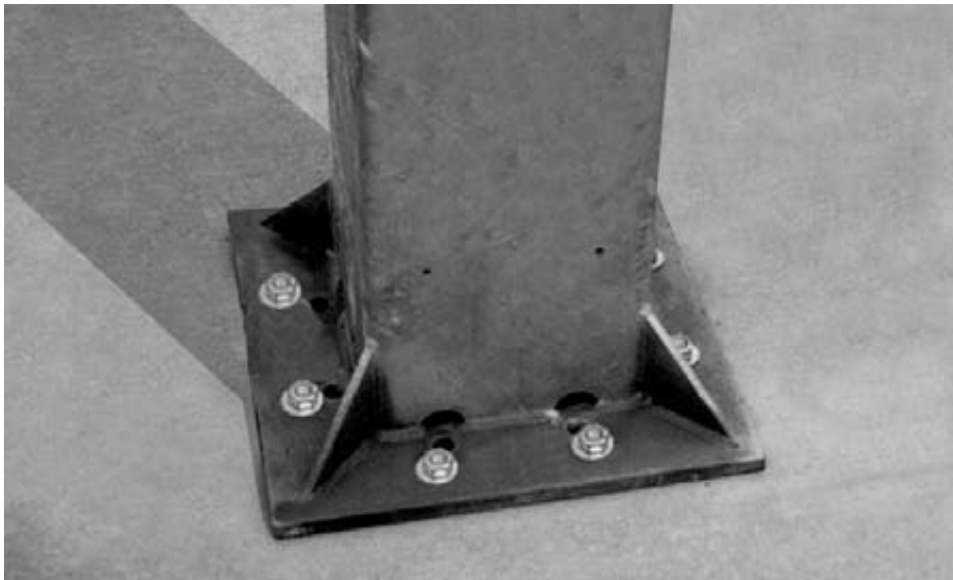
Figure 23 - Ground mount assembly attached to the foundation
