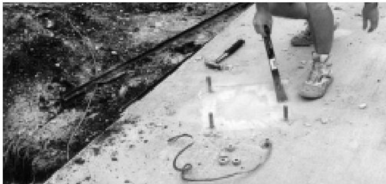
Figure 1-3: Scraping Foundation Pads
