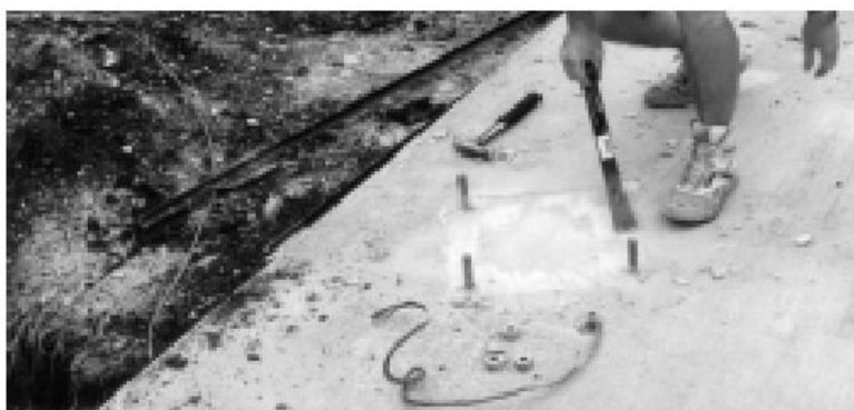
Figure 1-3: Scraping Foundation Pads
