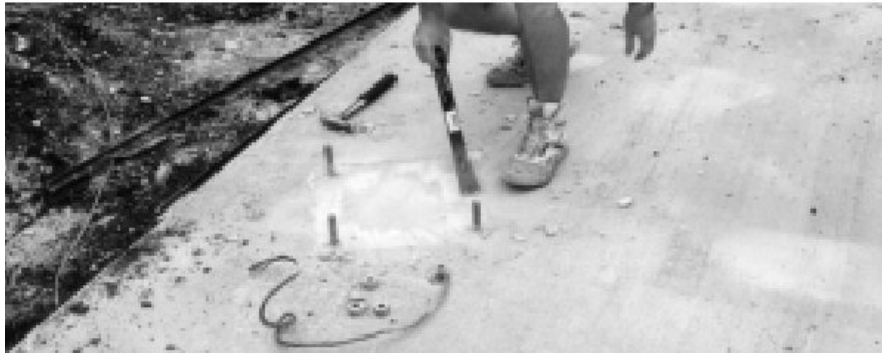
Figure 1-3: Scraping Foundation Pads
