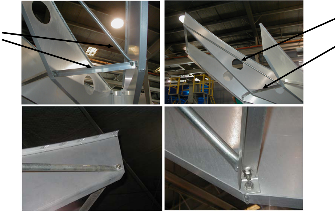
Figure 2-25. Lacing Between Radial #3 and Radial #4
