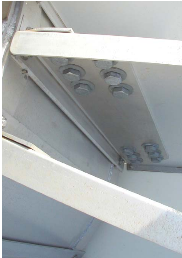
Figure 2-30. Install Radial Beam Stiffener
