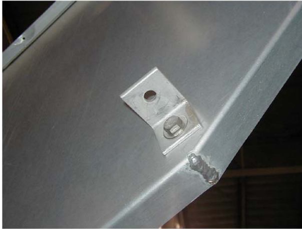
Figure 2-23. Angle Clips on Radials
