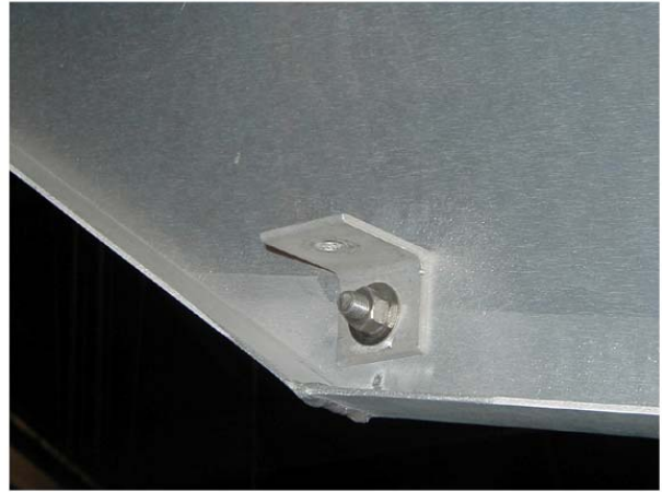
Figure 2-23. Angle Clips on Radials
