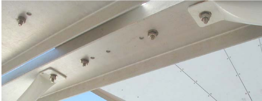
Figure 2-40. Install Feed Support Kit
