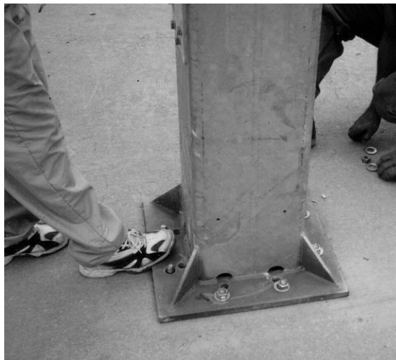
Figure 3-8a: Ground Mount Assembly Base Hardware
