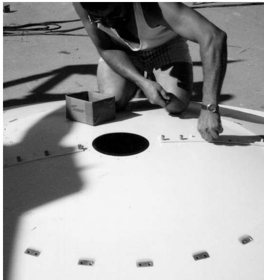
Figure 3-32: Seam Bolt Insertions
