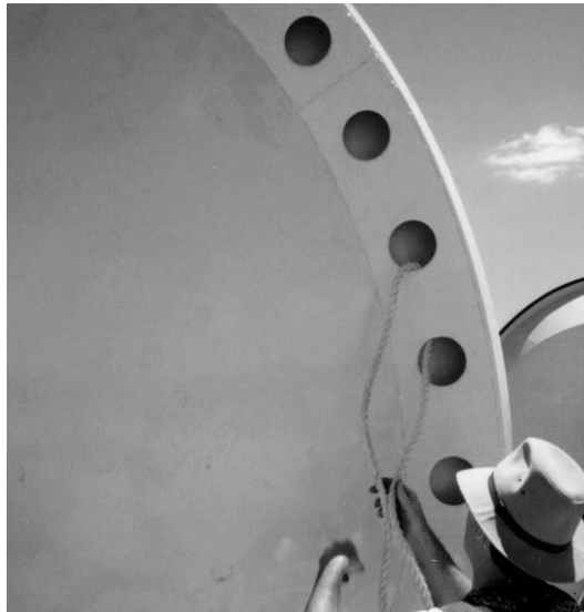
Figure 3-43: Safety Rope Tag Lines
