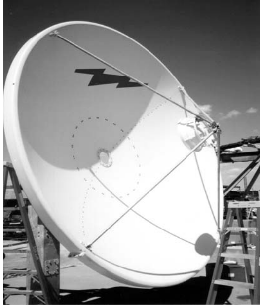
Figure 3-51: Installed Subreflector
