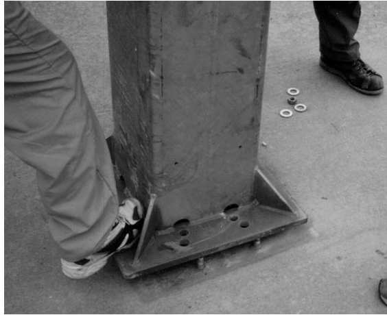
Figure 3-7: Mount Alignment/Adjustment
