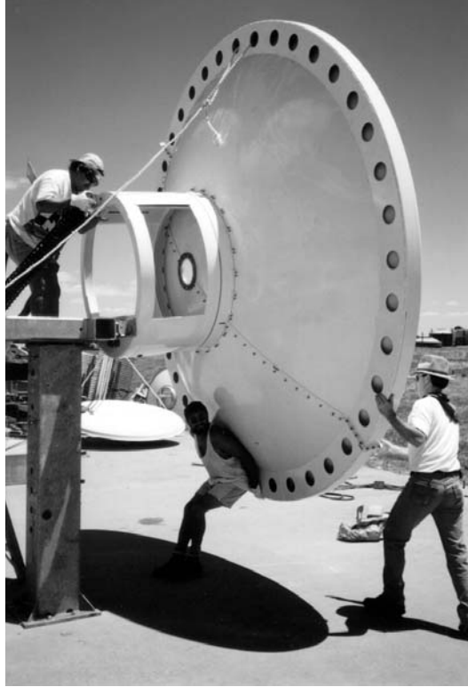
Figure 3-49: Elevation Jack/Enclosure Attachment
