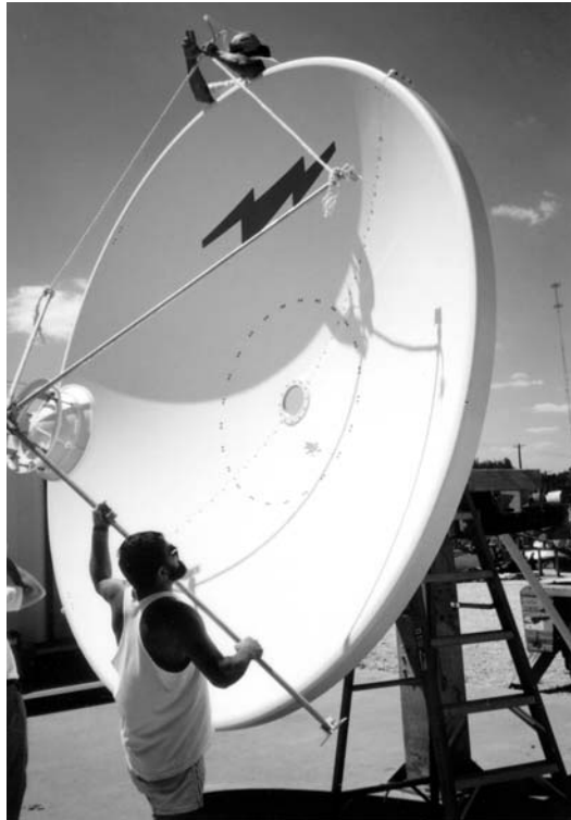
Figure 3-54b: Subreflector Attachment
