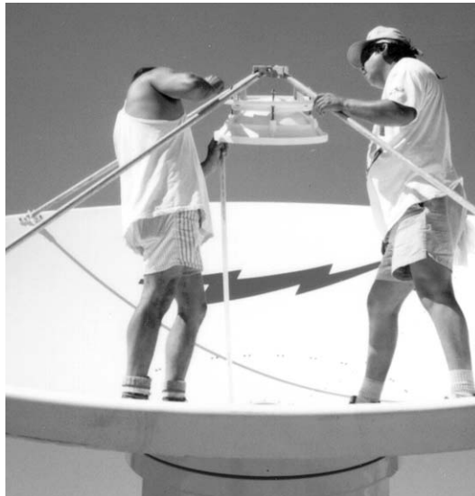
Figure 3-55: Subreflector Alignment
