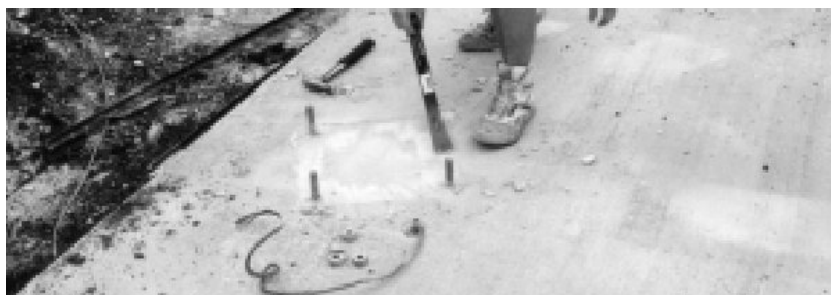
Figure 1-3: Scraping Foundation Pads
