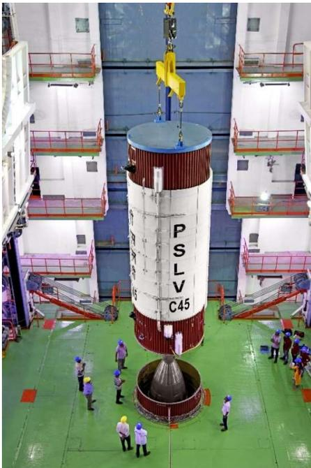
Hoisting of PSLV-C45 liquid second stage during vehicle integration
