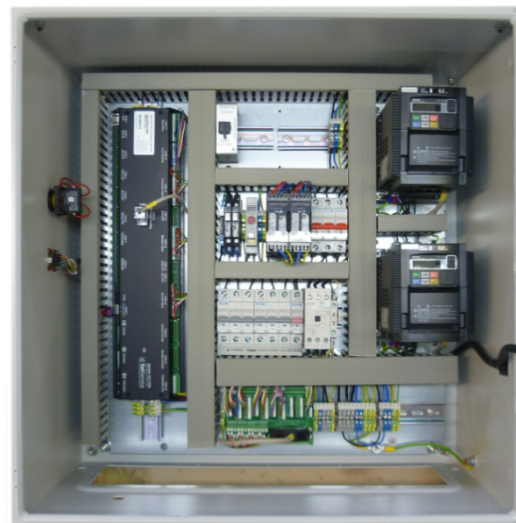
ACU-ODU-AC-DS, standard with 3kW inverters
