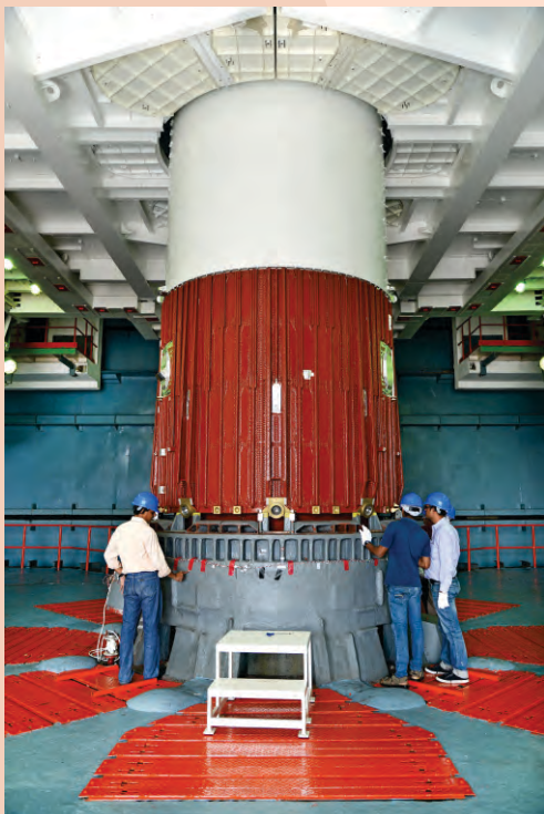
Placement of Nozzle End Segment of PSLV-C27 first stage over Launch Pedestal in progress
