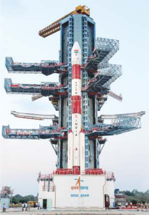
PSLV-C32 at the Second Launch Pad
