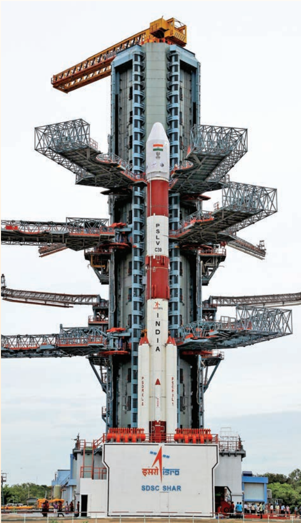
PSLV-C39 at the Second Launch Pad
