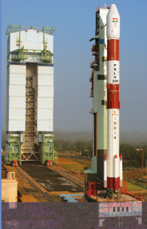
PSLV-C21 at the First Launch Pad
