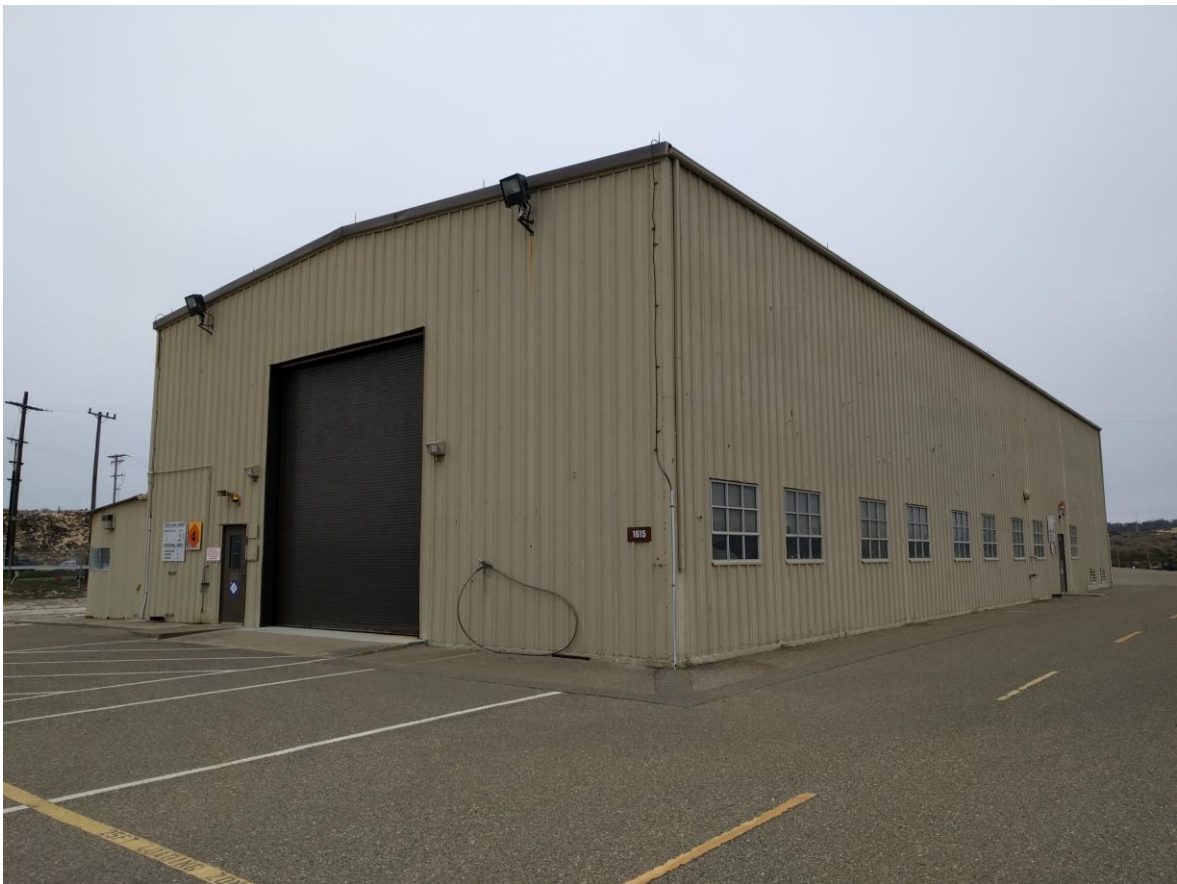
FIGURE 26 VAFB Horizontal Integration Facility
