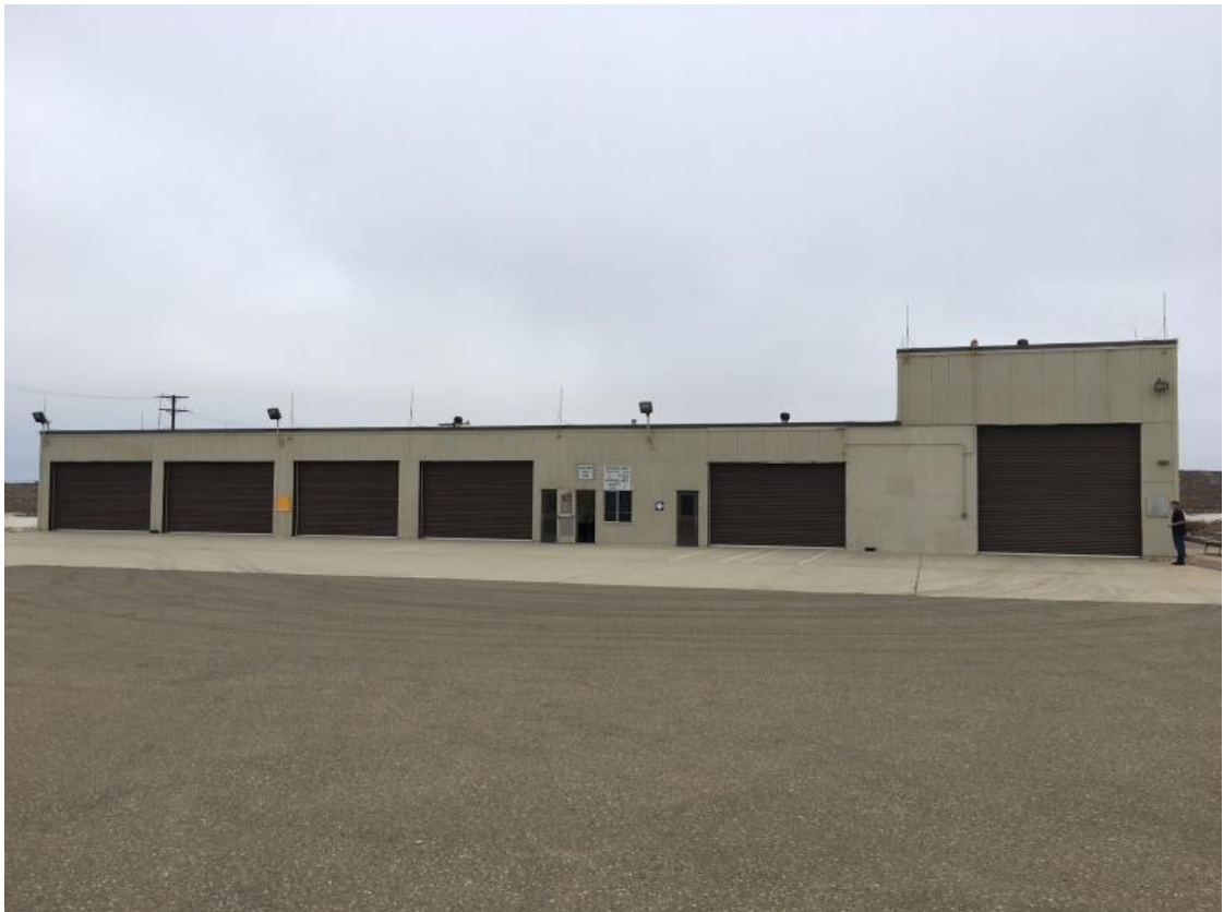
FIGURE 27 VAFB Payload Processing Facility
