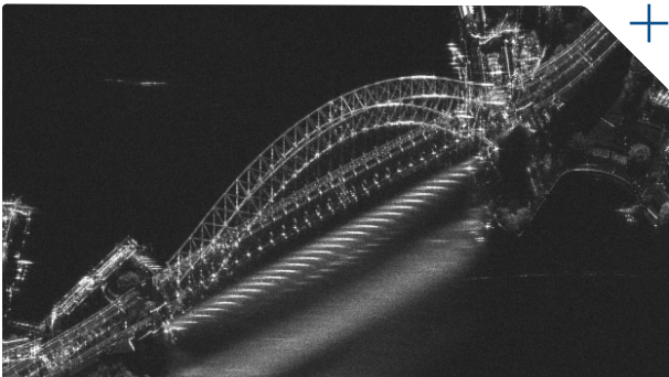
Sydney Harbour Bridge
